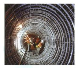
Nuovinox Stainless composite rebar with carbon steel core for construction.
